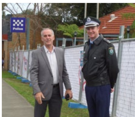
Greg and Lake Macquarie Local Area Commander Brett Greentree take a last look at the old Morisset Station before demolition.
